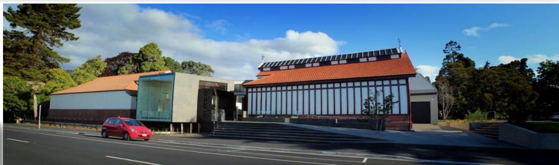
New Suter building Photographed by Eiji Toyokawa
